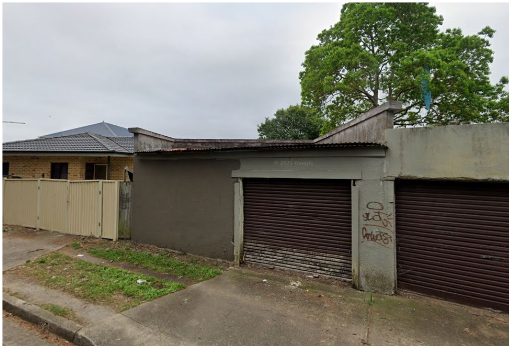
Figure 5 View of the existing garage from the rear of the site.
